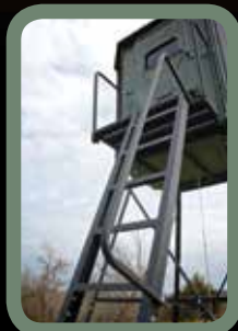
Sturdy Ladder & Platform Rails
