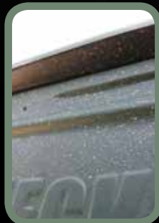
Drip Edges on Roof & Windows
